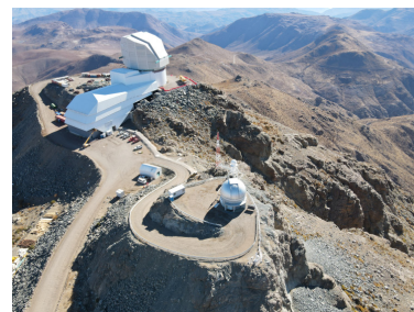
Figure 2: July, 2021 drone photo of the Rubin Observatory summit facility (provided by Dome Surveyor, Oscar Rivera) showing advancement to near 100% on the dome cladding completion as well as closure of the louvers, rear door, and shutters. Sublocation: Cerro Pachón, Chile. Credit: Rubin Obs/NSF/AURA
